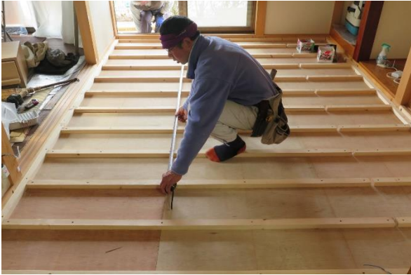
Remove the "Tatami" and apply Joists
