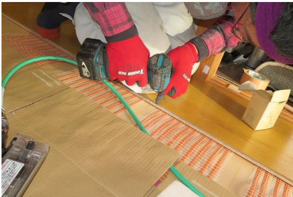
Parquet Flooring Placement & Screw panels on designated spaces
