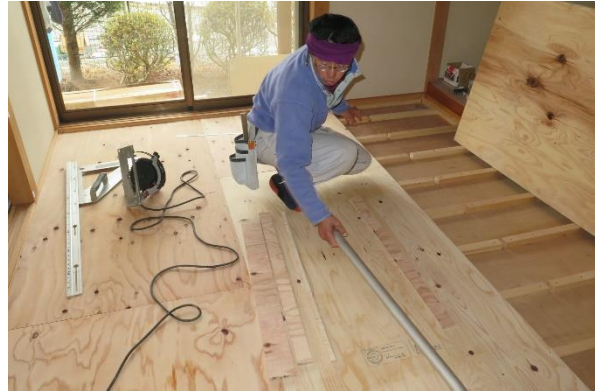
Install the Plywood Surface to cover Joists
