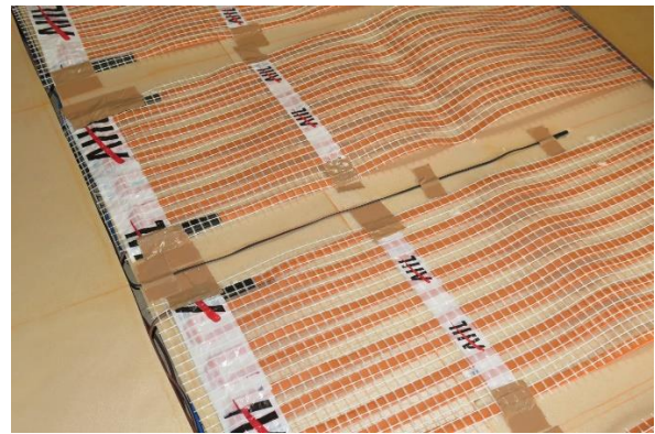
Floor Temperature Sensor placement
