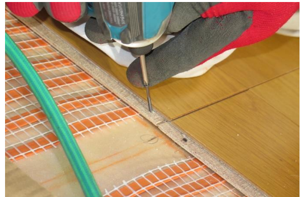
Parquet Flooring Placement & Screw panels on designated spaces
