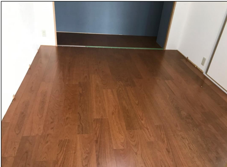
Applied parquet flooring
