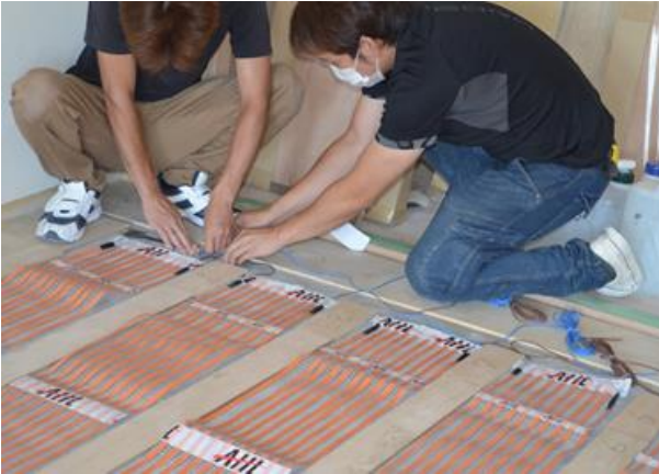
Wiring the cold leads
