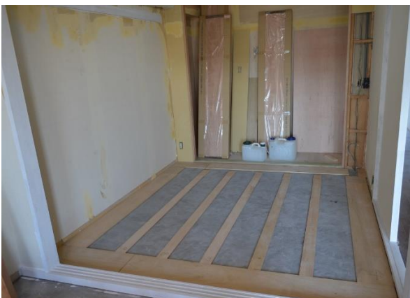
Preparation of underlayer insulation
