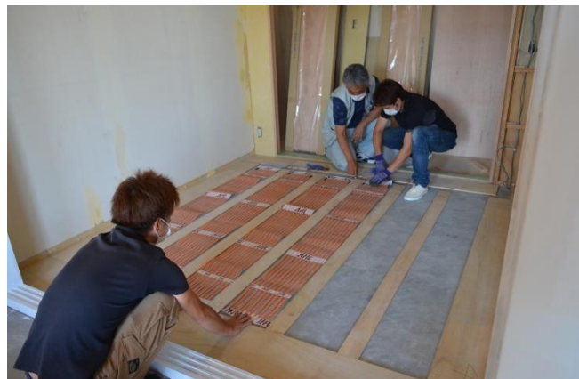
Laying out the customized heating mats
