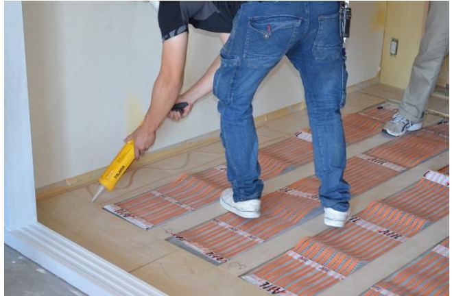
Dispensing adhesive substance for top plywood cover
