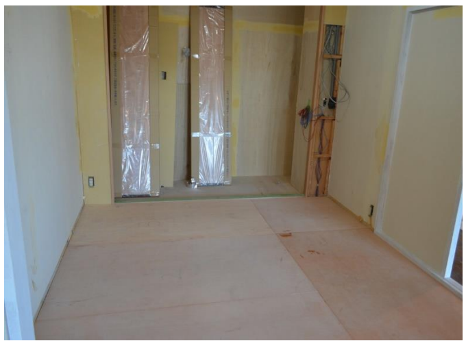
Top cover mounting completion
